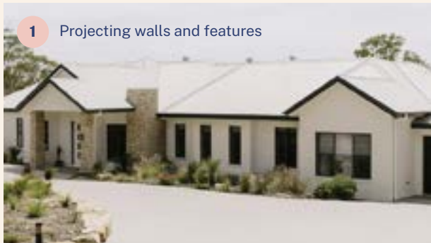
Image supplied by Macdonald Jones Homes
